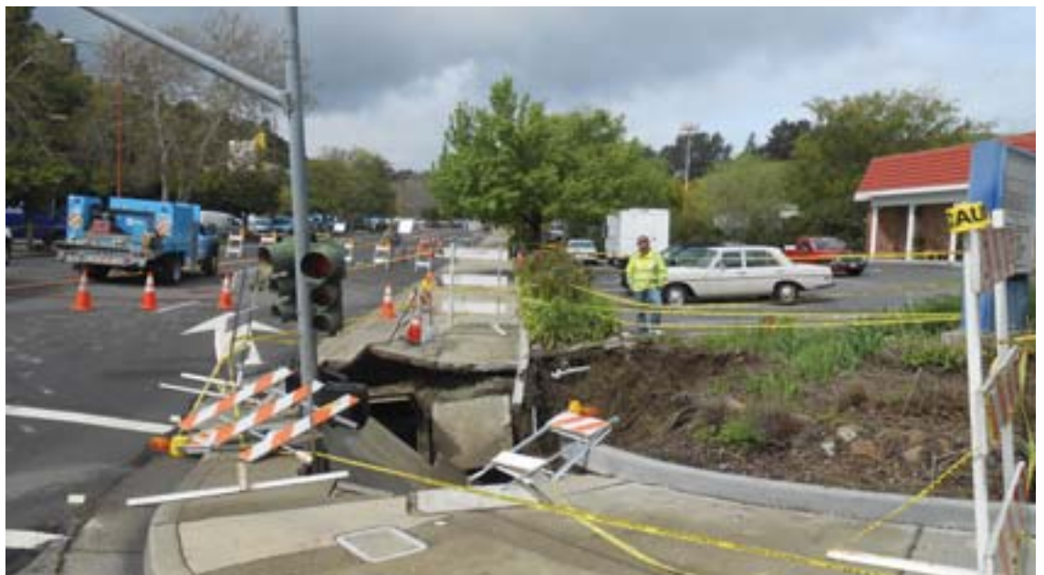
This sinkhole developed in March 2016 Photo provided
